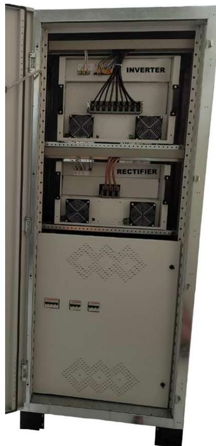
Figure 1.1. Power Modul Type Three Phase UPS\_33
